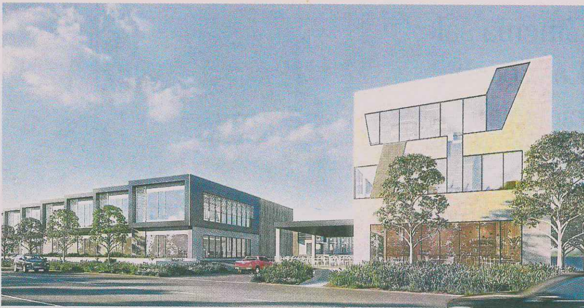
The $40 million Industria Nunawading will comprise warehouses and offices.
